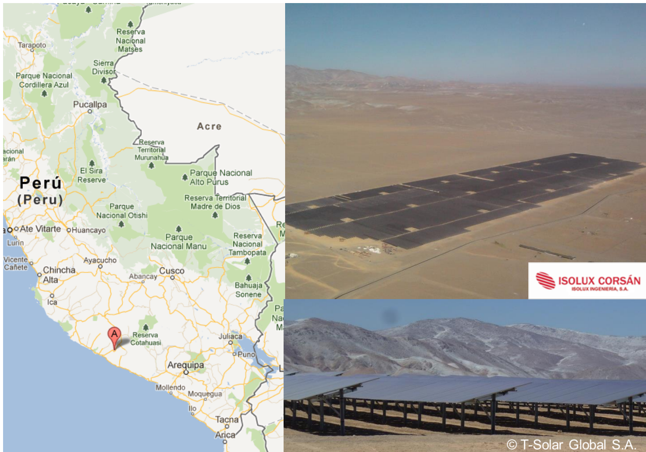
Figure 23: Approx. 50 000 T-Solar modules are installed in one of the two 22 MW PV plants in Peru. Here is shown the Repartición site near Arequipa in the south of Peru (marked by the letter A in the left side map).
